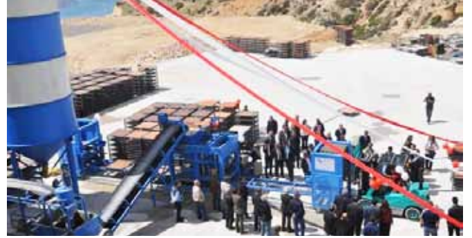
Türkiye - ZIM8 Beton Parke ve Blok Üretim Tesisi Turkey - ZIM8 Concrete Pavers and Block Production Facility
