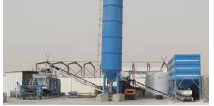
Katar - ZIM1025 Beton Parke ve Blok Üretim Tesisi Qatar - ZIM1025 Concrete Pavers and Block Production Facility
